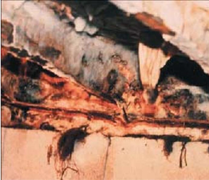
Figure 2: Damage to Wood from moisture
